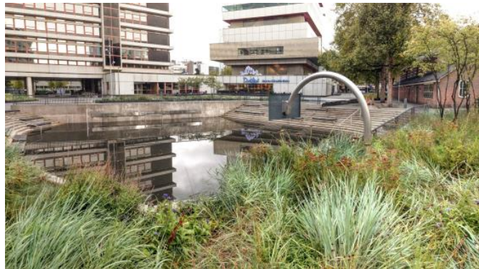
Figure 1: Benthemplein Water Square in Rotterdam – Climate-Adaptive Rainwater Storage and Public Space
